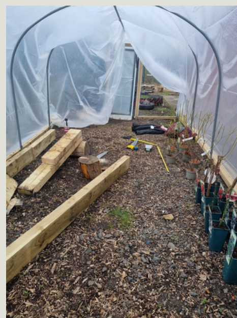
A New Larger Poly Tunnel Under Construction
